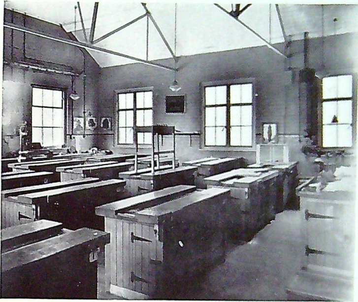
WOODWORK AND METALWORK SHOP
